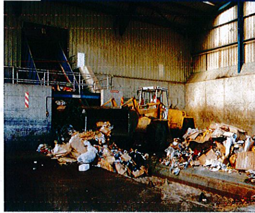
Infeed conveyor to a municipal solid waste processing facility (UK)
